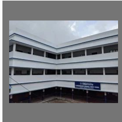
School Building Construction Service
