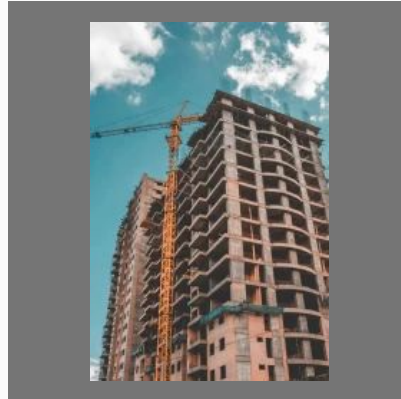
Multi Story Building Construction Service
