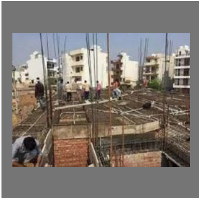
Commercial Building Construction Service
